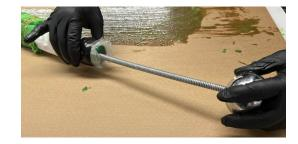
Insert prepared point repair packer into pipe.
