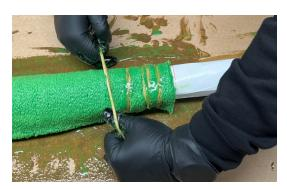
• After end caps side has been secured, start applying rubber bands every 10-15 cm (4-6").
