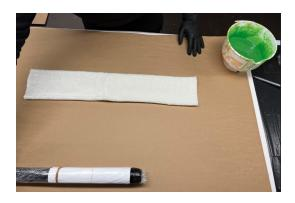
After resin is mixed according to the instructions, pour a portion on the surface of the patch material.
